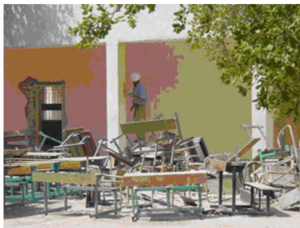
Repairing schools in Iraq
