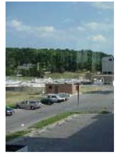
View from the Control Room
