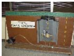
A typical water connection.
